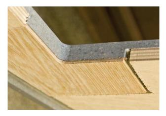
Tube steel, angle iron and wood are acceptable support materials (additional information in Support section). Particleboard and equivalent products are not acceptable as support or underlayment materials. Figures 7, 8, and 9 show support structures of tube steel, angle iron, and wood. In each set of diagrams, Figure A shows support for a cutout corner with the high-strength corner reinforcement block and Figure B shows support for the underlayment between the corner blocks.
